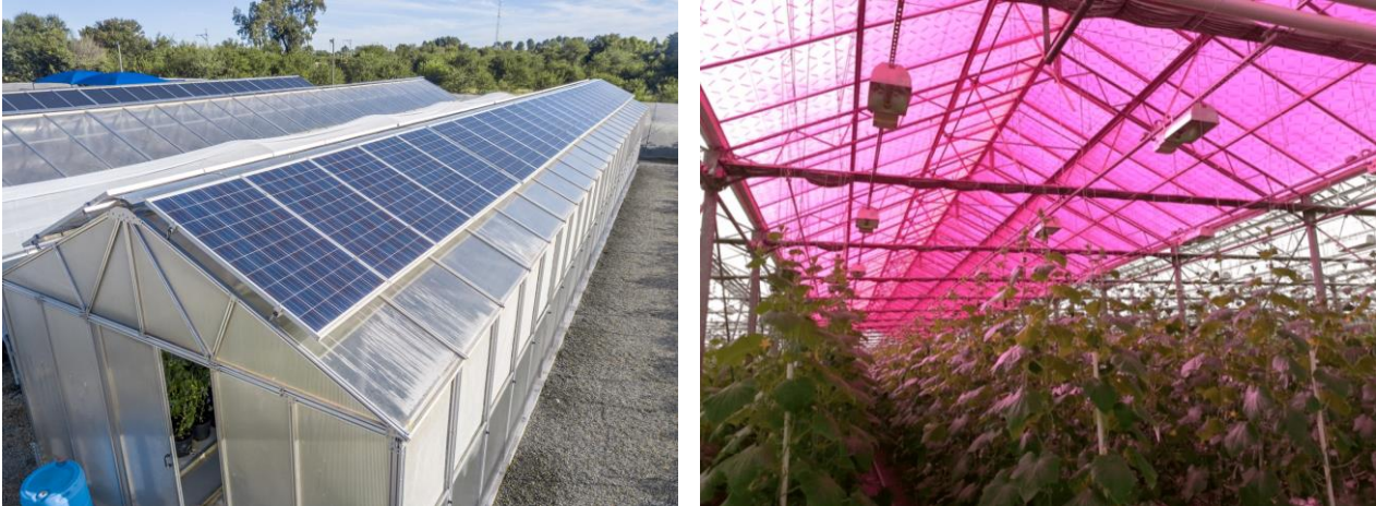
Fig. 1 Example of greenhouse with conventional PV (right) and colored transparent PV (left)
