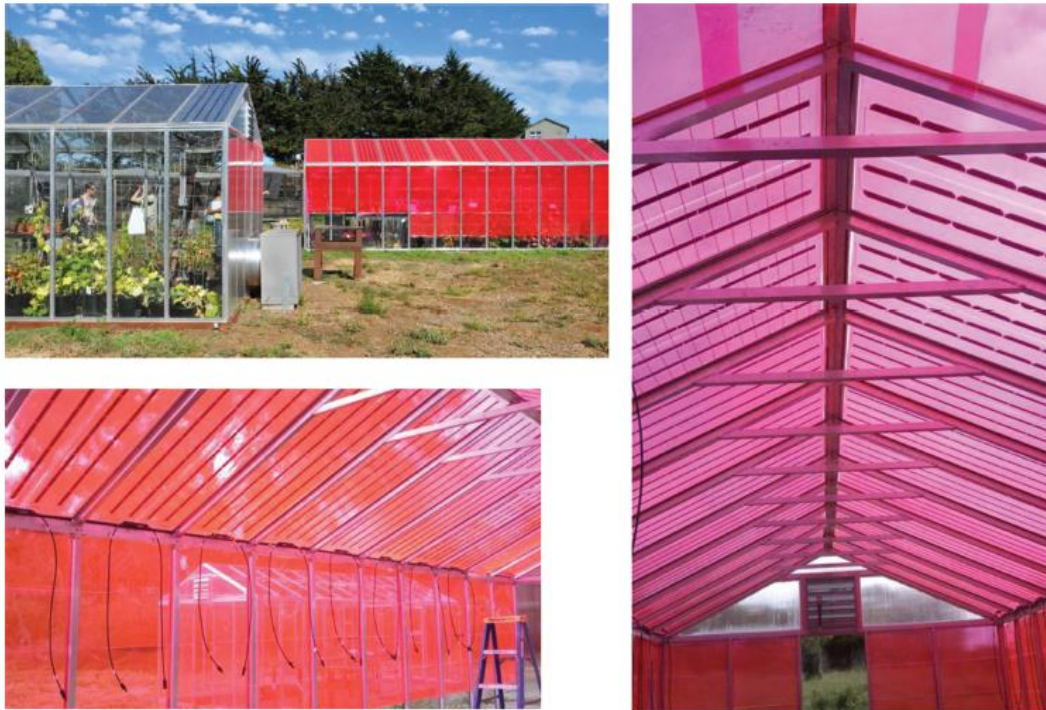
Fig. 4 Glasshouse constructed with Wavelength Selective Photovoltaic panels, at the University of California Santa Cruz Arboretum.
